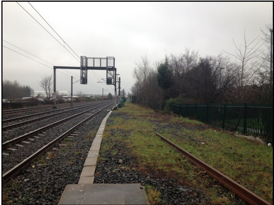
Figure 36: View from South Drive side decision point looking towards Hebburn Station (photograph provided by Network Rail) – Network Rail’s ALCRM report records the sighting distance as 317 metres.
