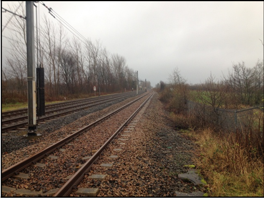
Figure 37: View from Riverside Park side decision point looking towards Pelaw Station (photograph provided by Network Rail) – Network Rail’s ALCRM report records the sighting distance as 585 metres. TSP Projects believe this photograph and sighting distance was taken before the crossing signage was relocated to the decision point. Currently, the sighting at the decision point is obscured by the crossing signage.
