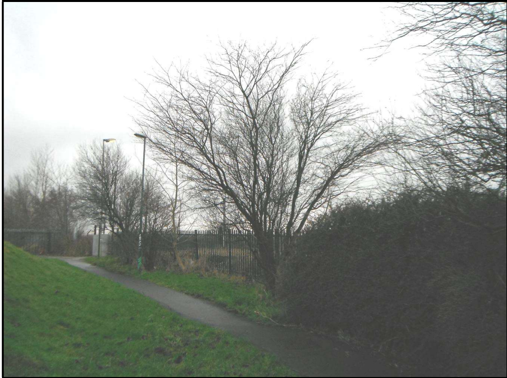
Figure 10: Pedestrian access towards the crossing from Woodvale Drive. The asphalt path provides good underfoot conditions and is illuminated by street lighting provided by South Tyneside Council. The railway boundary fence appears to be in good condition and of a suitable height/type to deter unwanted access.
