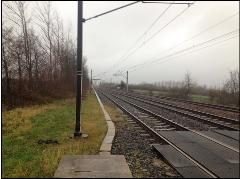
Figure 35: View from South Drive side decision point looking towards Pelaw Station (photograph provided by Network Rail) – Network Rail’s ALCRM report records the sighting distance as 780 metres.
