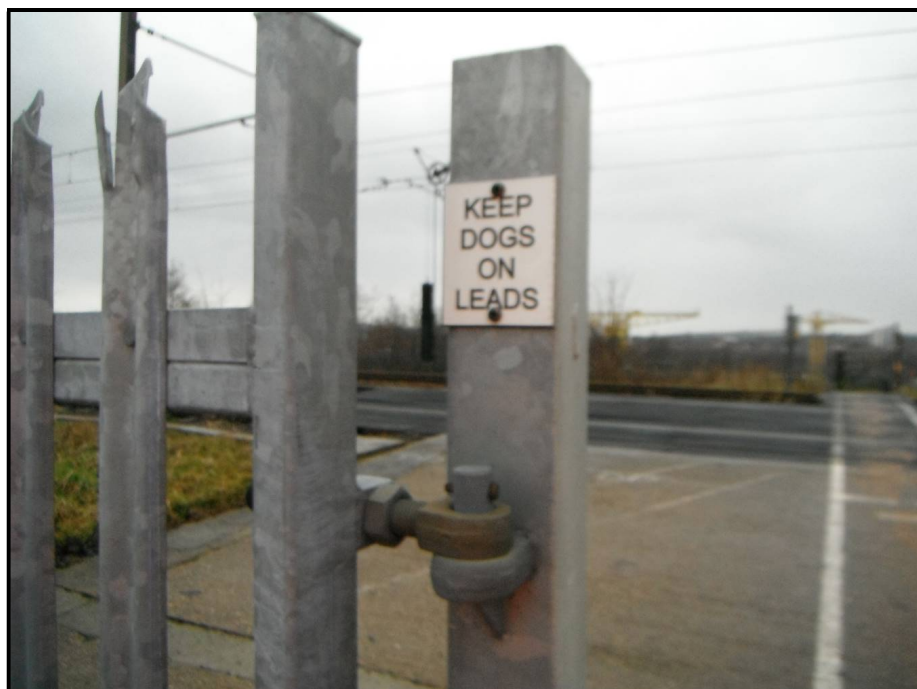
Figure 17: The existing sign infers a high usage of the crossing by dog walkers. During the site visit, a dog on an extendable lead walked off the decking and into the four foot of the Network Rail line. The 9 day Census of Rail and Pedestrian Users concluded that an average of 63 dog walkers use the crossing per day (maximum of 106 on Monday 4 th February 2017).
