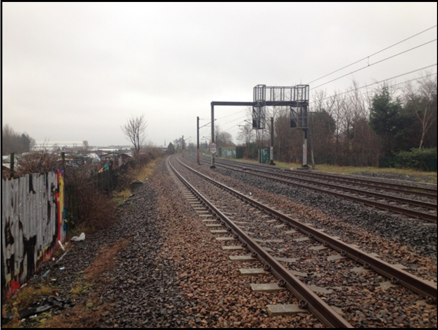
Figure 38: View from Riverside Park side decision point looking towards Hebburn Station (photograph provided by Network Rail) – Network Rail’s ALCRM report records the sighting distance as 417 metres.
