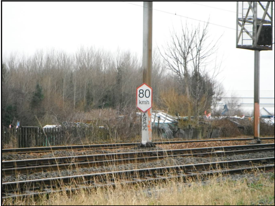
Figure 21: The presence of graffiti below the speed board in the ten foot shows that there are instances of trespass, most likely accessed from the crossing itself. No anti-trespass guards are installed at the crossing to act as a deterrent.
